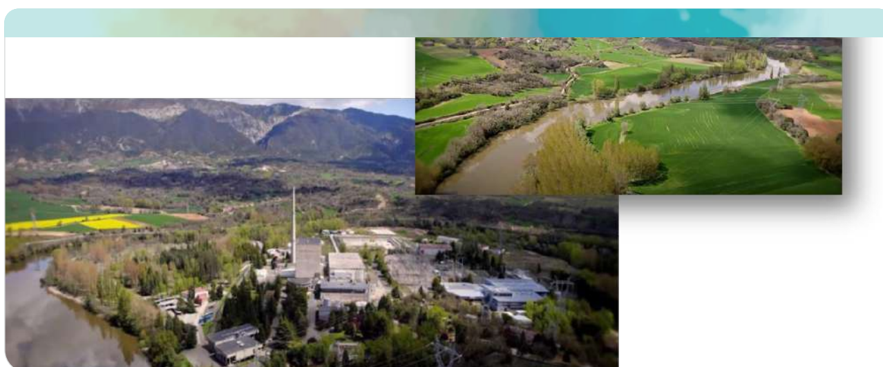
Figure 3. Santa María de Garoña Nuclear Power Plant (current and future forecast)
