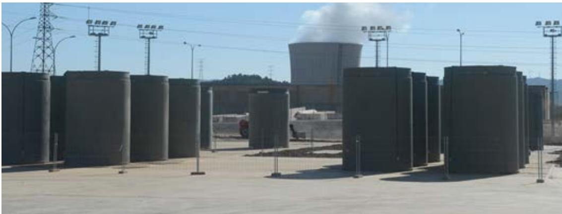
Image of the Ascó Nuclear Power Plant ATI.
