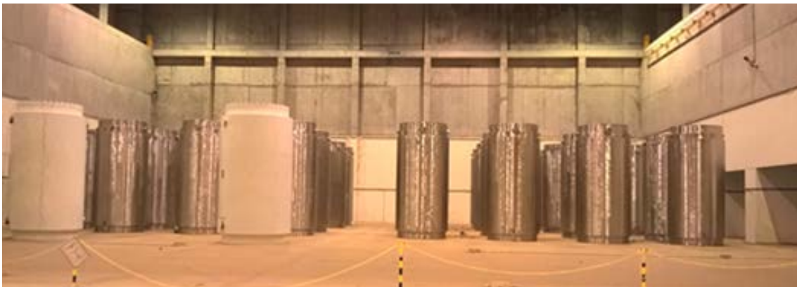
Image of Trillo Nuclear Power Plant ATI.
