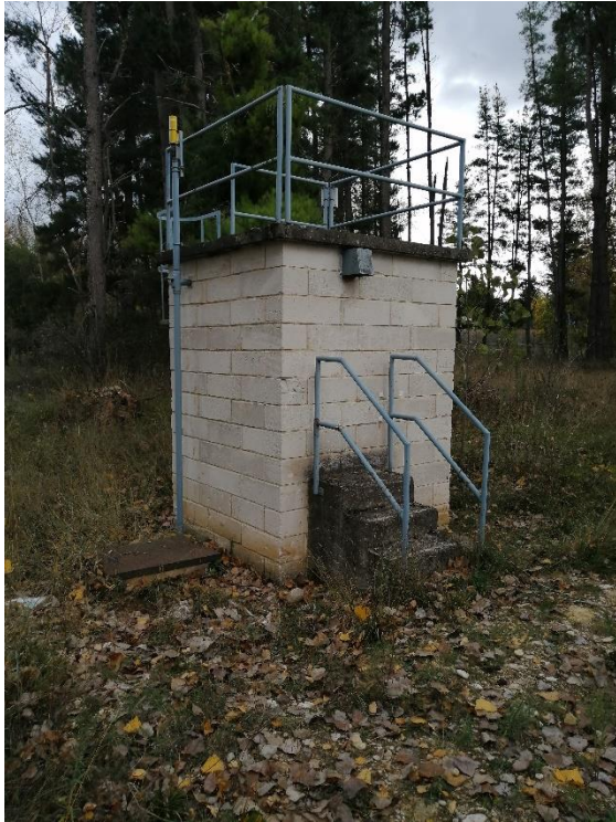
Figure 6. On-site monitoring location 3
