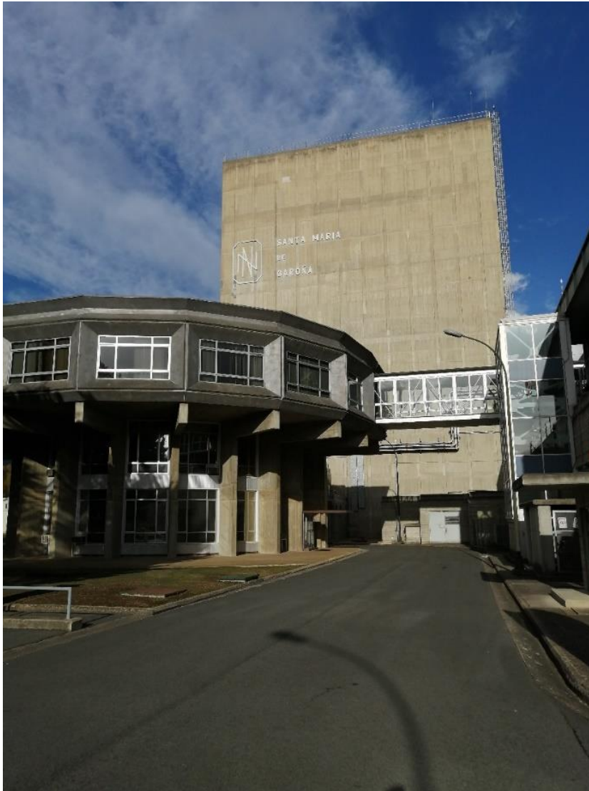
Figure 1. Garoña nuclear power plant
