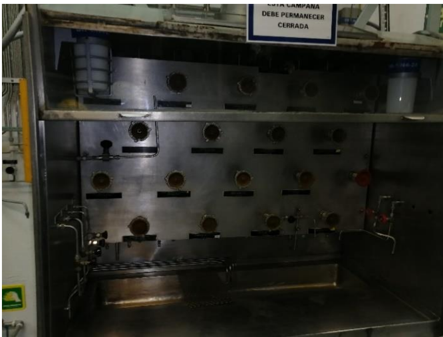
Figure 19. Liquid waste tank sampling cabinet
