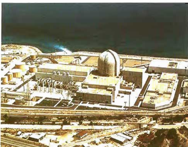
Central nuclear Vandellós II.
